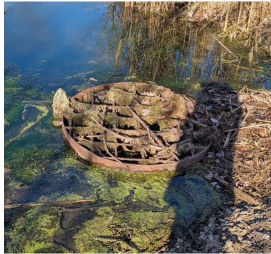
Figure 1: Drain in retention basin behind Creek Bend
